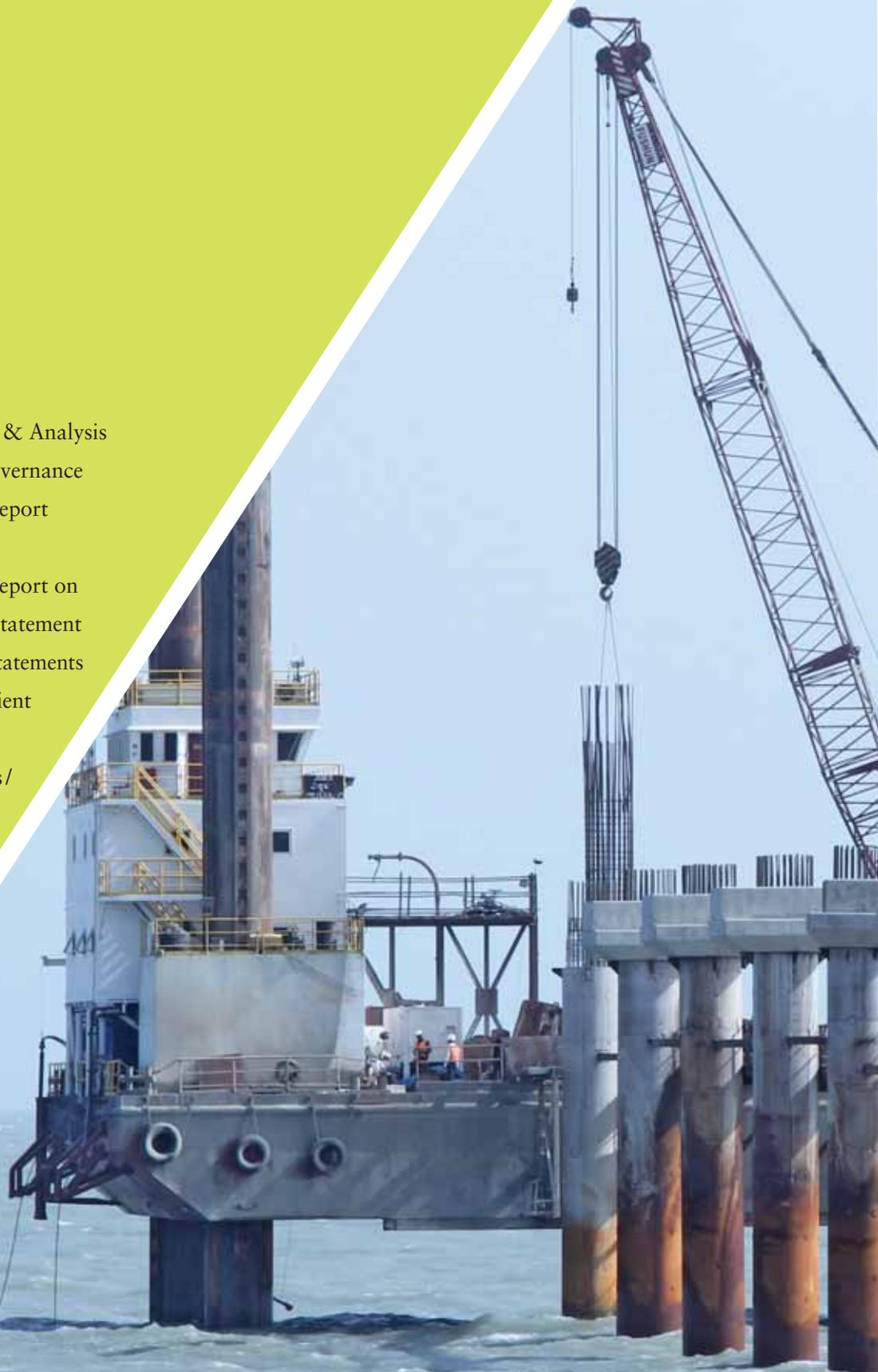
*Installation of 1600mm dia Bored Cast-in-Situ-piles in progress by Jack up Berge in open sea in Gulf of Kutch at Mundra for LNG Jetty Project for Adani Ports & SEZ Ltd.*
