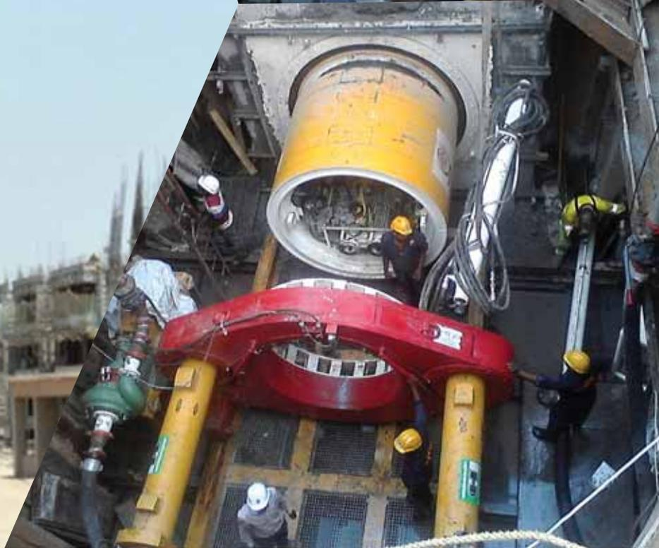
*Micro tunneling work in progress for laying of 1829 mm dia concrete
