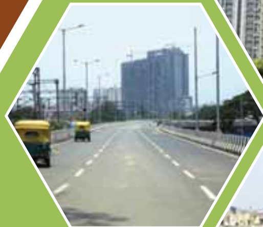
View from Bangalore Station of Completed Flyover at Okalipuram
