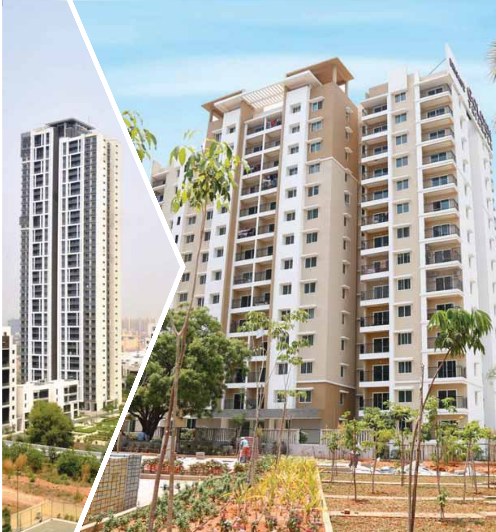
Construction of Brigade Golden Triangle Apartment Complex at Bengaluru
