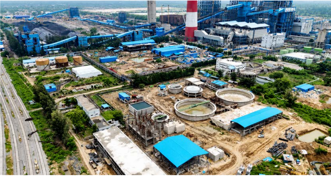
Water Treatment Plant for 2X800 MW Power Plant for Adani Power Project Raigarh, Chhattisgarh
