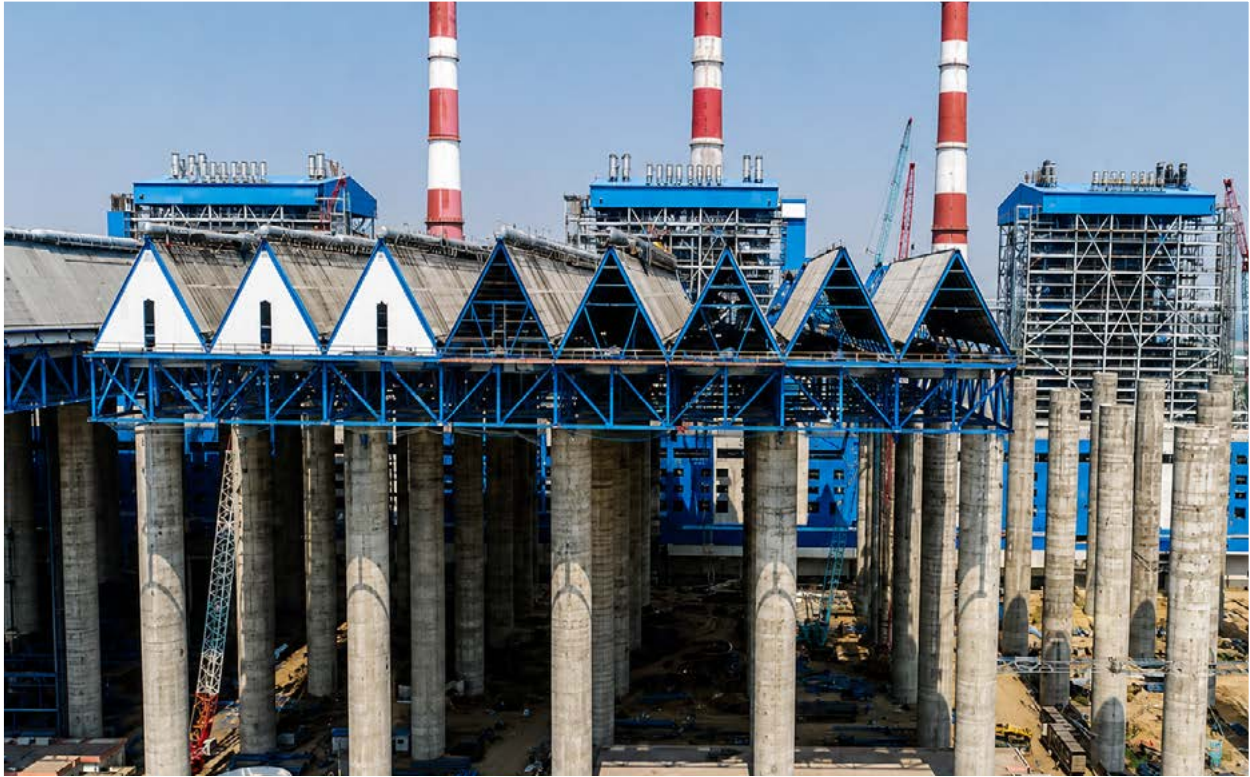
Air Cooled Condenser 5.4Mtr Dia and 54.8 Mtr Height RCC Hollow Column using Slipform Technology for NTPC 3X660 MW Thermal Power Plant at North Karanpura, Jharkhand.
