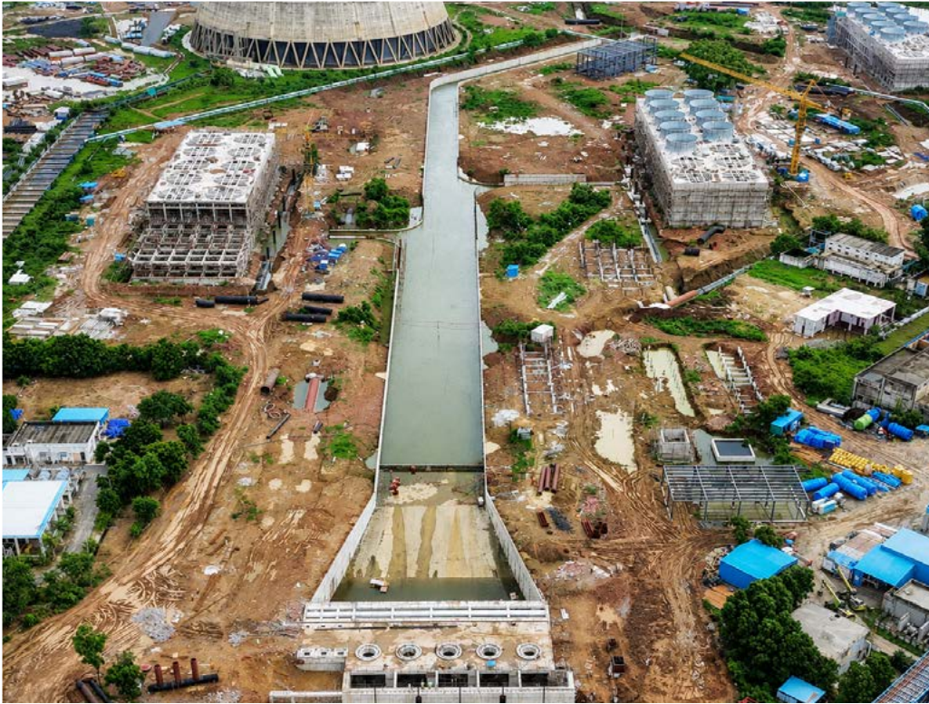
Circulating Water Pump House, Forebay & Circulating Water Channel for 2X800 MW Adani Power Project (PH-II) at Raigarh, Chhattisgarh
